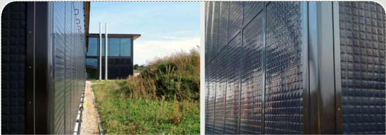
FIGURE 8: Partial view of a non-active facade. The stainless steel elements are visible below the windows of the upper floor (left).
