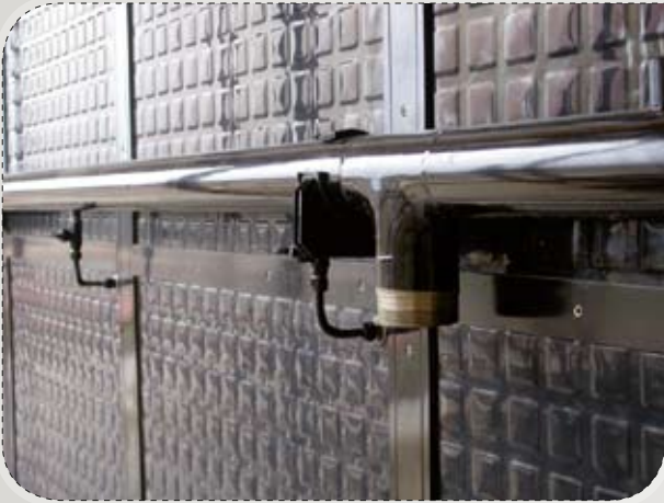
FIGURE 12: Close-up of the connection of the collectors to the upper tube for heat transfer fluid
