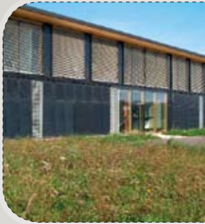
FIGURE 5: South facade with unglazed stainless steel solar collectors for floor heating and hot water. The connections between the absorber elements and the distribution pipes for the heat-transfer fluid are visible.
