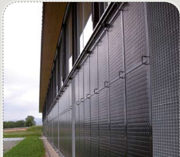
FIGURE 9: Details of the interconnection of the stainless steel collectors and connection to the upper tube for the heat transfer fluid
